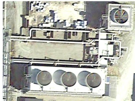
Plant cooling towers
