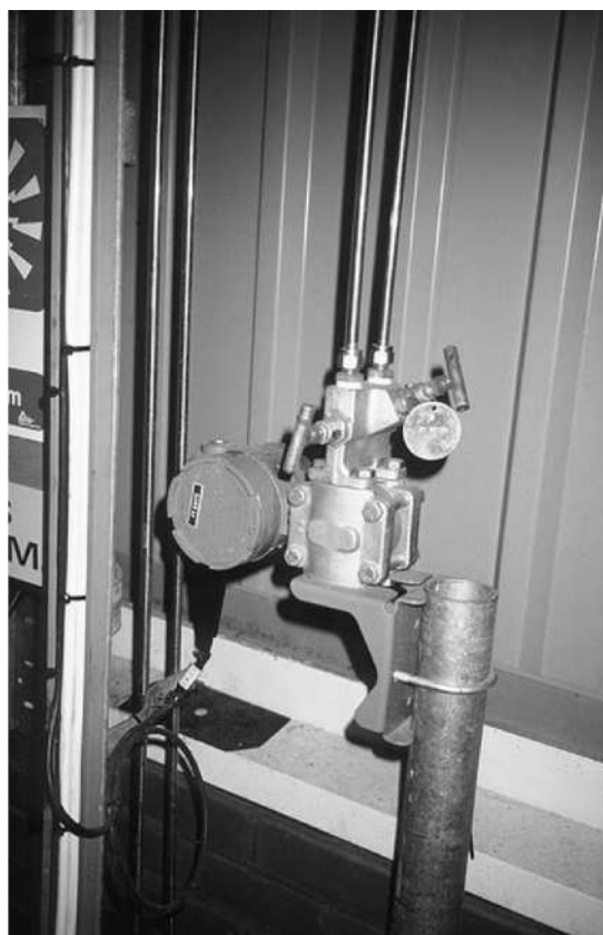
Picture 11.2 Installation showing dp cell, impulse lines, manifold and supports
