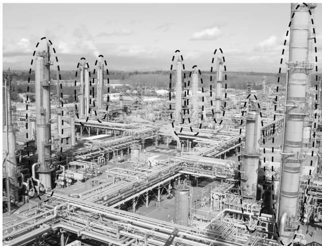
FIGURE 4.1 Refinery Landscape Dominated by Distillation Columns (Encircled by Dotted Ovals)
