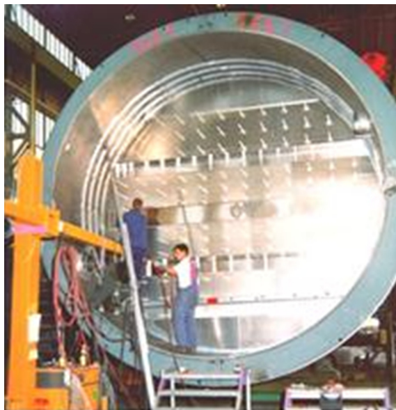
FIGURE 6.11 Photograph of the Installation of a Four-Path Sieve Tray in a Column that is 4.9 m in Diameter.
