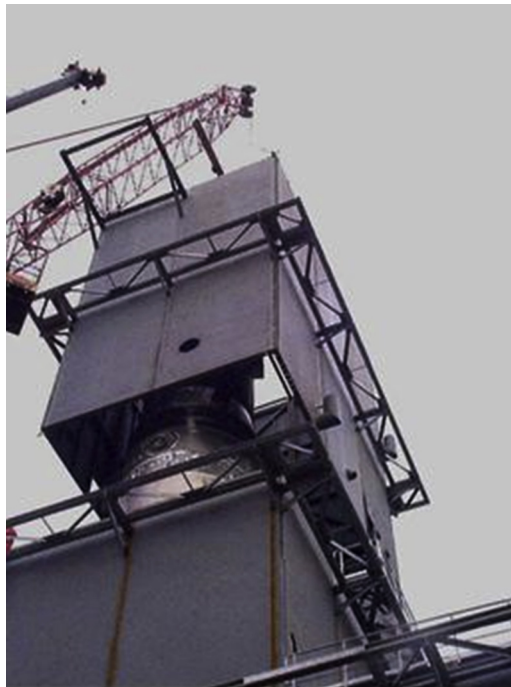
FIGURE 6.7 Coldbox Assembly of a Site-Erected Air Separation Unit.
