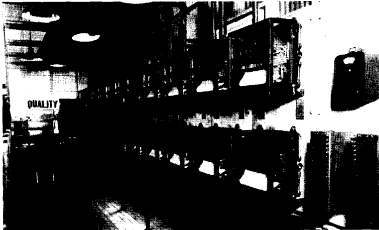
Fig. 2. A bank of Leeds & Northrup Company controllers installed in the hardening room of the Continental Motors Co., Muskegon, MI. The illustration is from [41].
