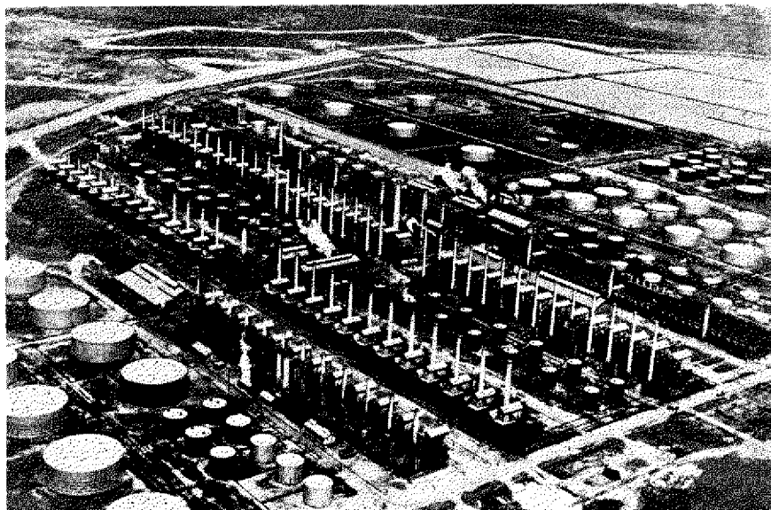
Installation of Holmes-Manley Vertical Stills at Port Arthur Works of the Texas Company
