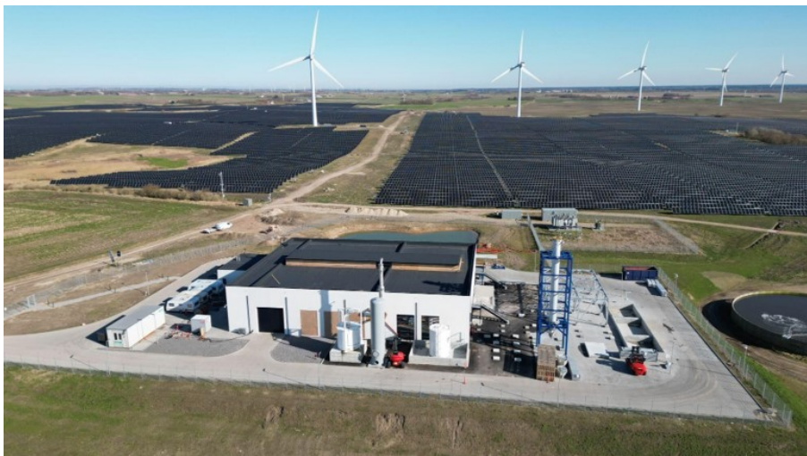
Figure 2.4: Air photograph of Skovgaard Energy's 10 MW PtA plant under construction in Ramme, Denmark.
