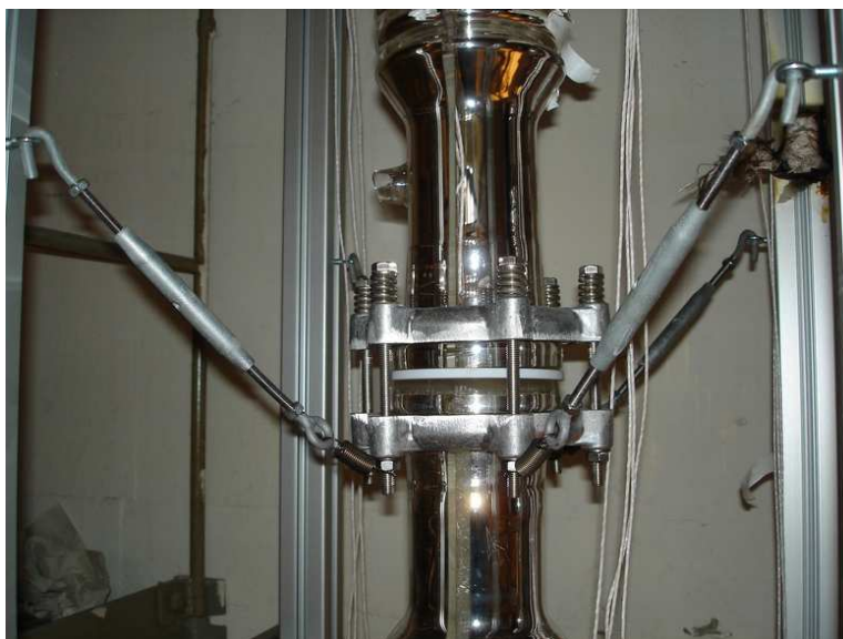
Figure 9.3: Springs and turnbuckles help centering the column and relieves pressure from the sections below
