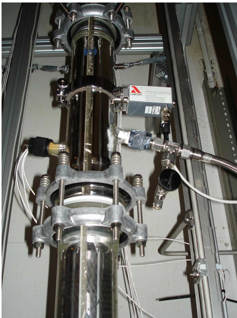
Figure 7.2: Side-stream product draw. Swinging funnel inside column section directs the liquid to the product line or as reflux.
