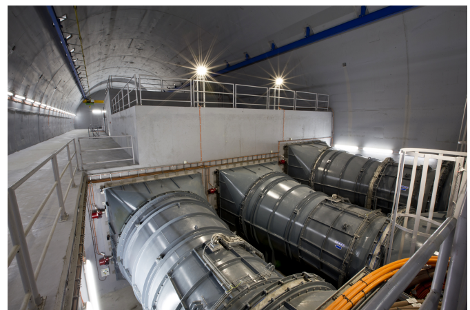
Figure 2: Ventilation machine room Letná including three axial fans for smoke extraction from the tunnel (2015) [11, 12].
