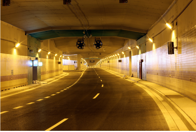
Figure 4: A pair of jet fans located at the ceiling of the tunnel. On the left, you can see the entrance ramp Prašný most. The photo was taken during the construction of the tunnel (February 2014) [11].
