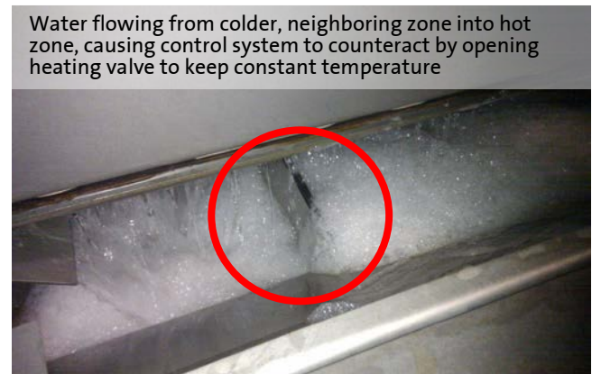
Fig. 7: Water overflow from one zone to another
