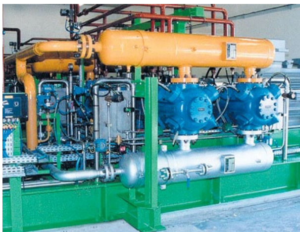
Fig. 1. An industrial two stage compressor, the two cylinders of stage one can be seen (blue)
