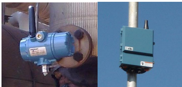
Fig 4. A WirelessHART sensor and gateway placement.
