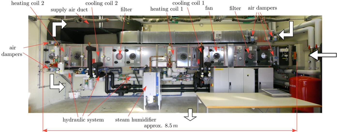
Fig. 1. Picture of the used HVAC test plant.
