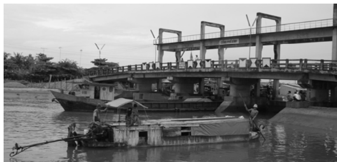
Figure 1 (a) – Sluice gate on a Mekong River estuary.
