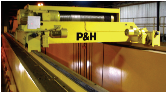
(b) Closeup of trolley.
