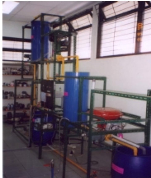
Fig. 6. View of the process mini-plant
