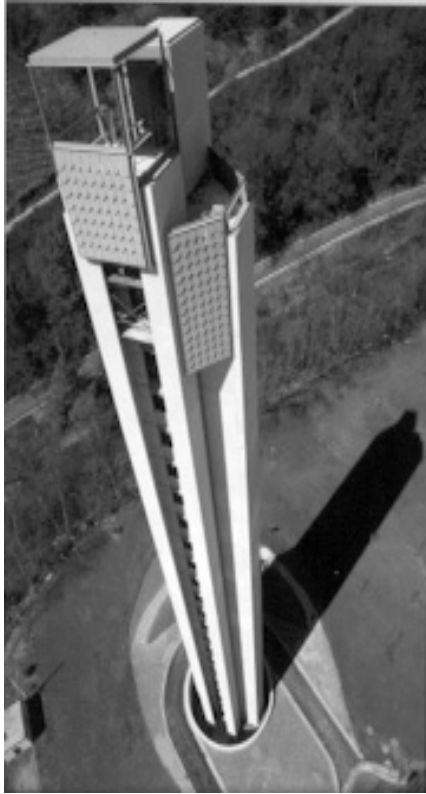
Fig. 1. View of the ORONA's ONDDI tower.
