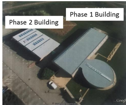
Figure 3. NEF Buildings Phase 1 and 2.
