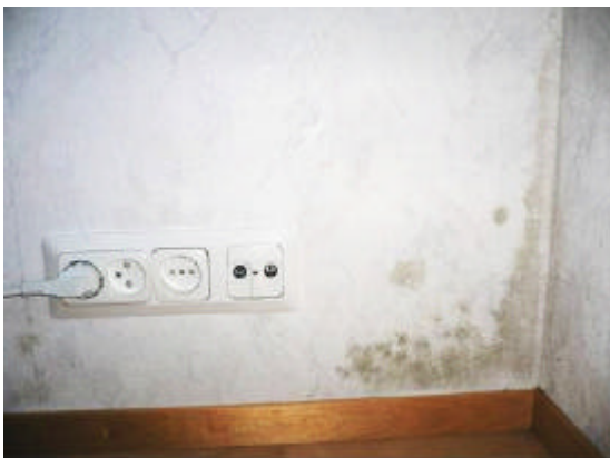
Fig 1. Photo of the corner having mildew stains.
