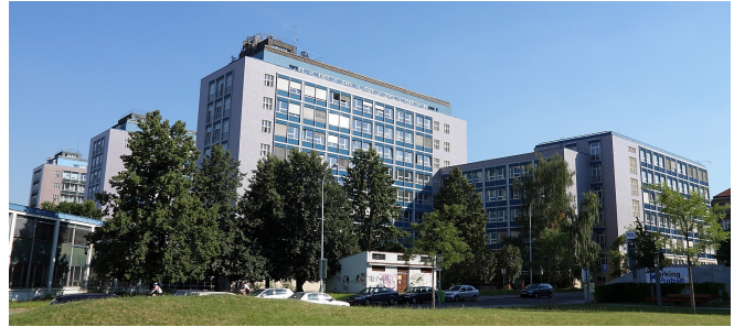
Fig. 1. Building of the Czech Technical University in Prague
