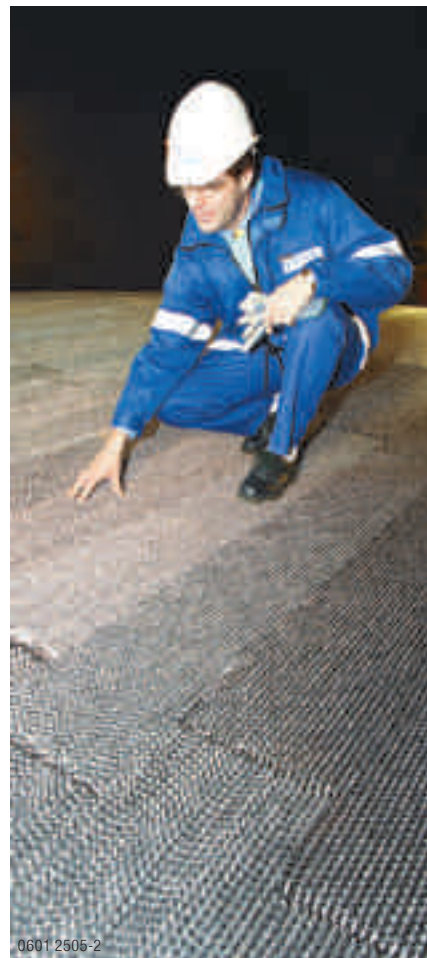
Inspecting packings after installation
