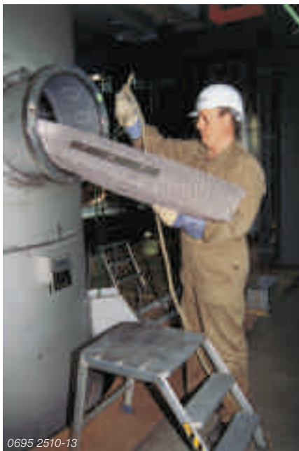
Installation of packing
