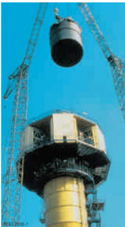
The column sleeve is lowered into the column with two cranes. Weight: 100 tons
