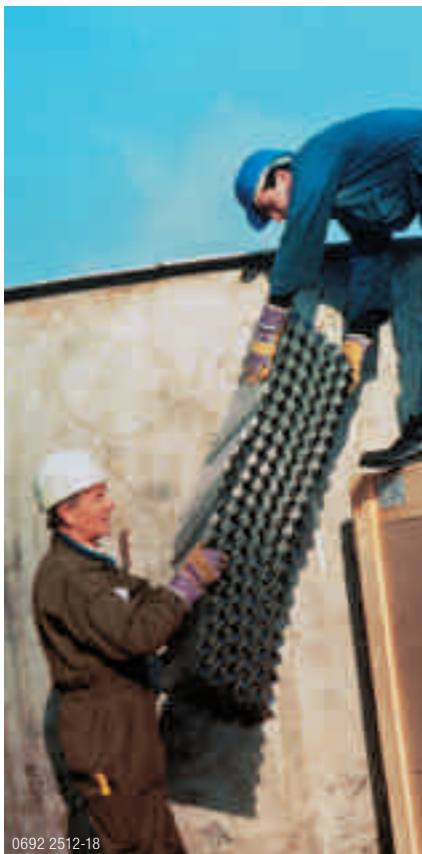
Revamping of a vacuum column with Mellapak
