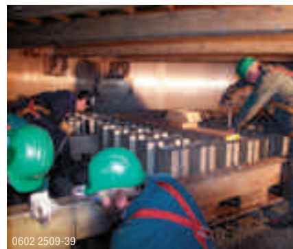
Installation of the liquid distributor
