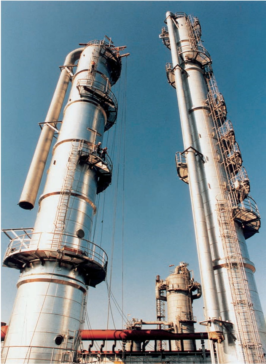
◀ Packed column DN 4000 during installation of Montz-Pak Type B1-250
