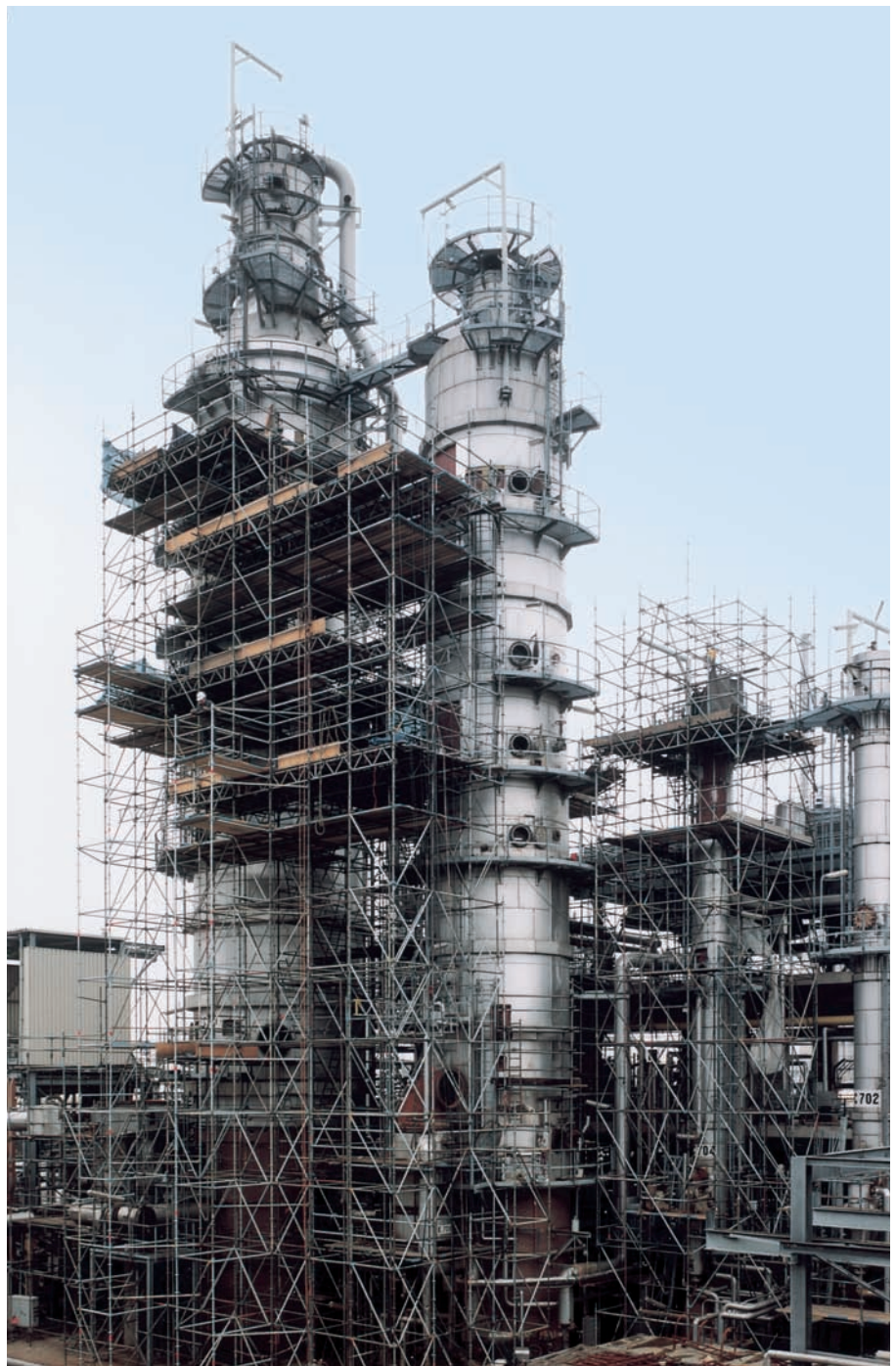
Two columns DN 5600 and DN 3800 during revamping with Montz-Paks
