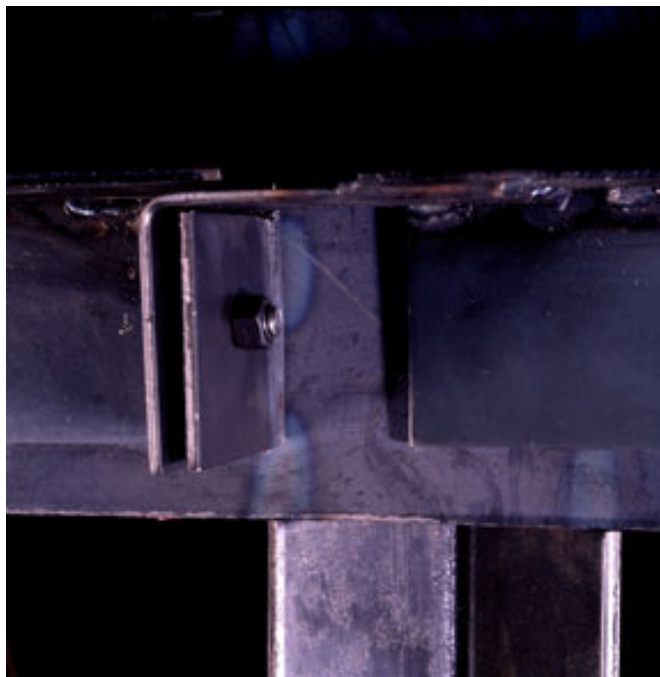
Figure 7. Close-up of Omni-Fit Expansion Ring
