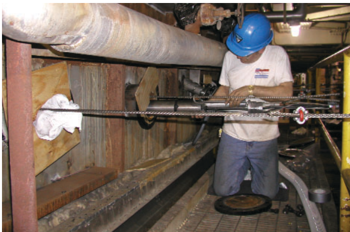
Insertion of the PDPA into a FGD scrubber.
