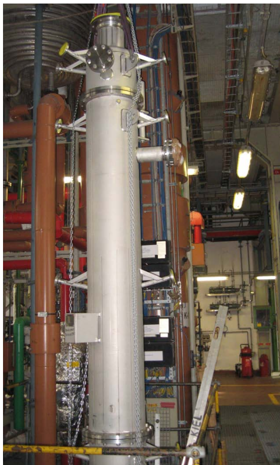
Figure 1: Installation of a new column for efficiency measurements at BASF, Ludwigshafen. The column body can be pivoted for easier installation of internals.
