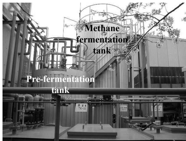
**Figure 5** The fermentation tanks
