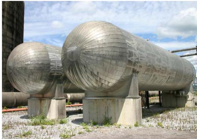
Representative **storage tanks for the working fluid and refrigerant**
