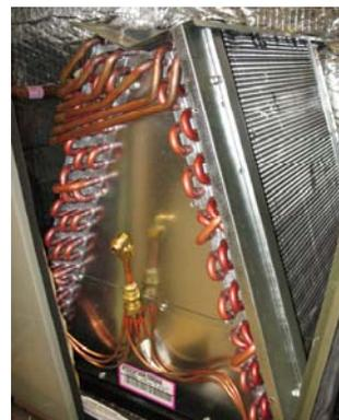
Figure 4: Actual heat exchanger with multiple distribution paths and varied geometry
