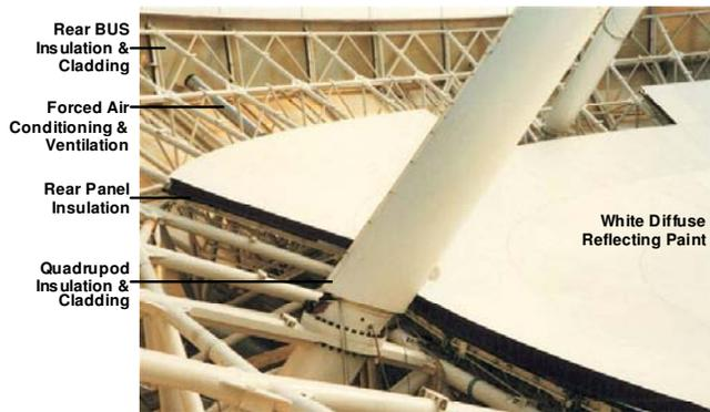
Figure XII-2 Thermal layout of the 30m MRT Spain reflector
