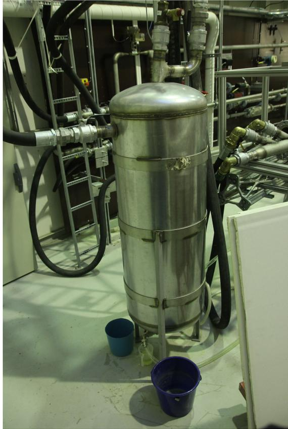
**Figure 3.4:** The buffer tank
