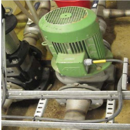
Figure 17: Water Centrifugal Pump
